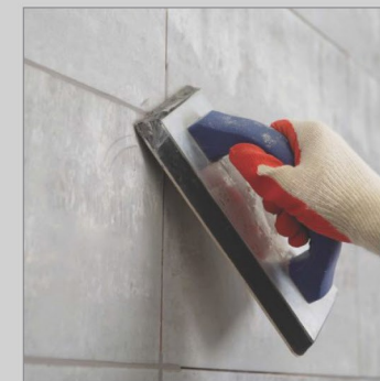
Joint Grouting
