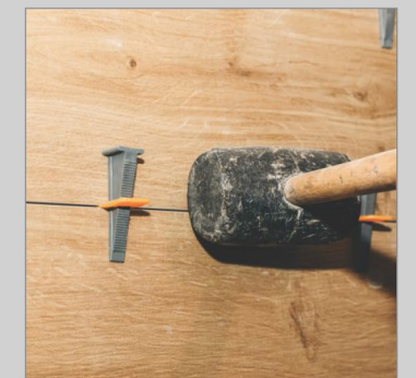
Remove Wedges Ones It Dry
