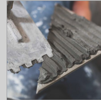
Cement Laying On Tile
